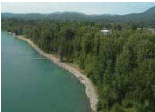
2004 bank stabilization, / Jerry Luther photo
